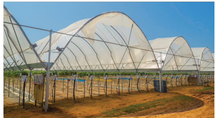
Figure 7. An example of a multi-bay high tunnel. Notice the uncovered support posts that allow for continuity throughout the space.
