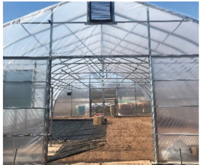
Figure 6. An example of a gothic-style greenhouse. Notice the height of the structure, allowing for tall vine crops to be grown in a more uniform environment the degree of structural support in the end walls. Photo credit: Talia Plaskett, Perennia
