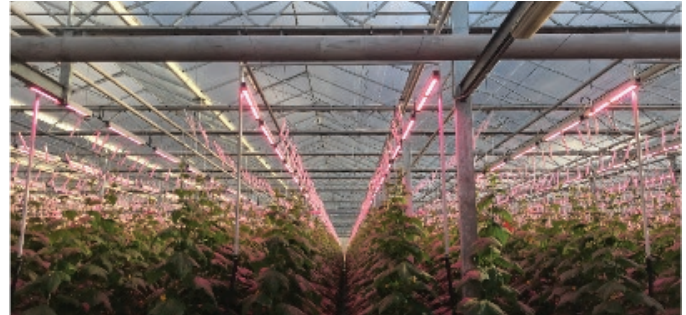
Figure 8. A greenhouse used to grow high-wire cucumbers. The addition of lights, in this case, was to allow for four-season production. Notice the thin profile of the lights, which reduces shadows cast on the crop from the overhead sun. Photo credit: Talia Plaskett, Perennia
