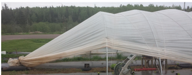
Figure 2. An image of a large caterpillar tunnel, with the end-to-end plastic typically seen in this style of tunnel. The structure's basic components are seen here – anchor which the end of the plastic is secured around, the hoops that support the plastic, the plastic itself, and the tie-down material used to hold the plastic against the metal frame. Photo credit: https://multisheltersolutions.com/applications/hanley-caterpillar-greenhouses/
