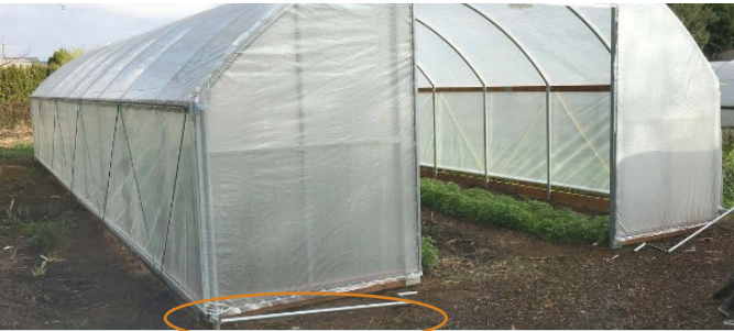
Figure 5. An example of a Quonset-style high tunnel. Notice the extra reinforcement inside the structure compared to the basic caterpillar structure. Pictured on the ground on the left side is a crank used to adjust the size of the side vents. Picture credit: https://www.greenhouseht.com/quonset-greenhouse
